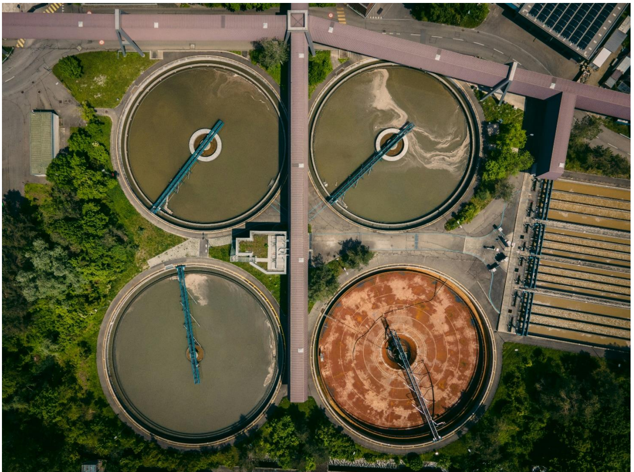
Figure 1: Sewage treatment plant © Patrick Federi, Unsplash
