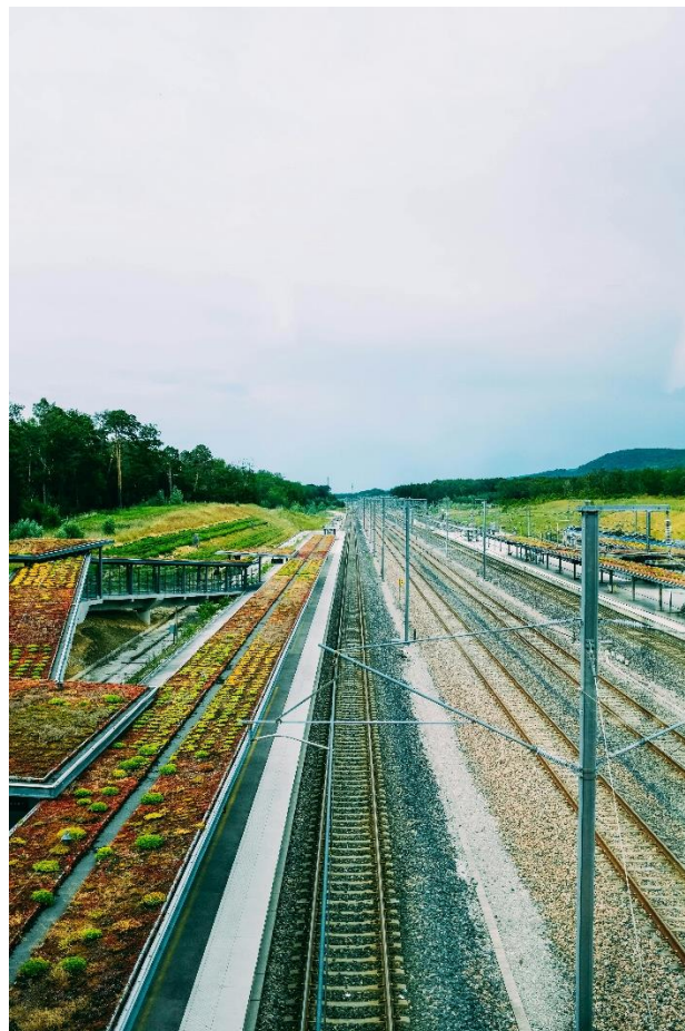
Figure 4. Green roofing along a railway line, an example of green infrastructure © Adrien Olichon, Pexels
