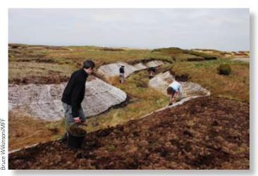
Plug planting into gully side stabilised by geo-textile
