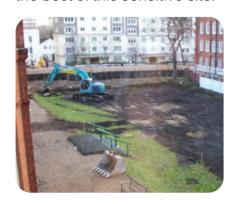
Heavy machinery moved on to the site as builders Durkan Pudelek began a complex two-year project to build the new extension on a very tight building site. A huge piling rig sank supports to a depth of 15 to 20 metres.
