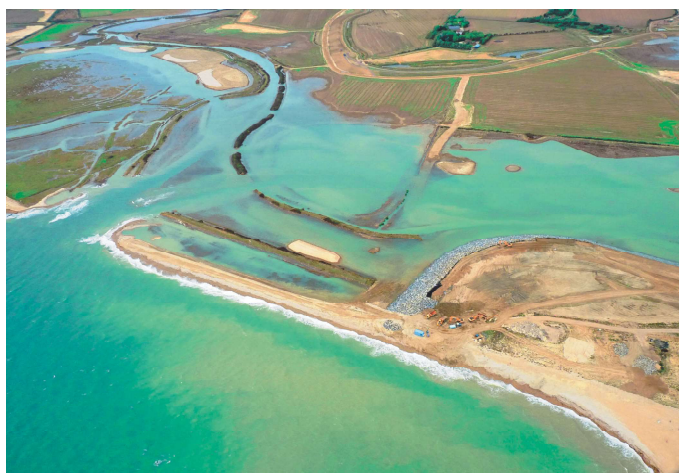
Medmerry Realignment: New Civil Engineer
