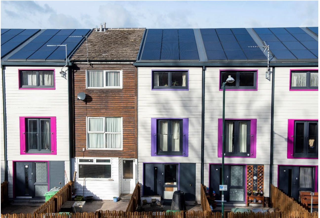
Figure 2 one house remains to be retrofitted in Nottingham © Tracey Whitefoot Energiesprong
