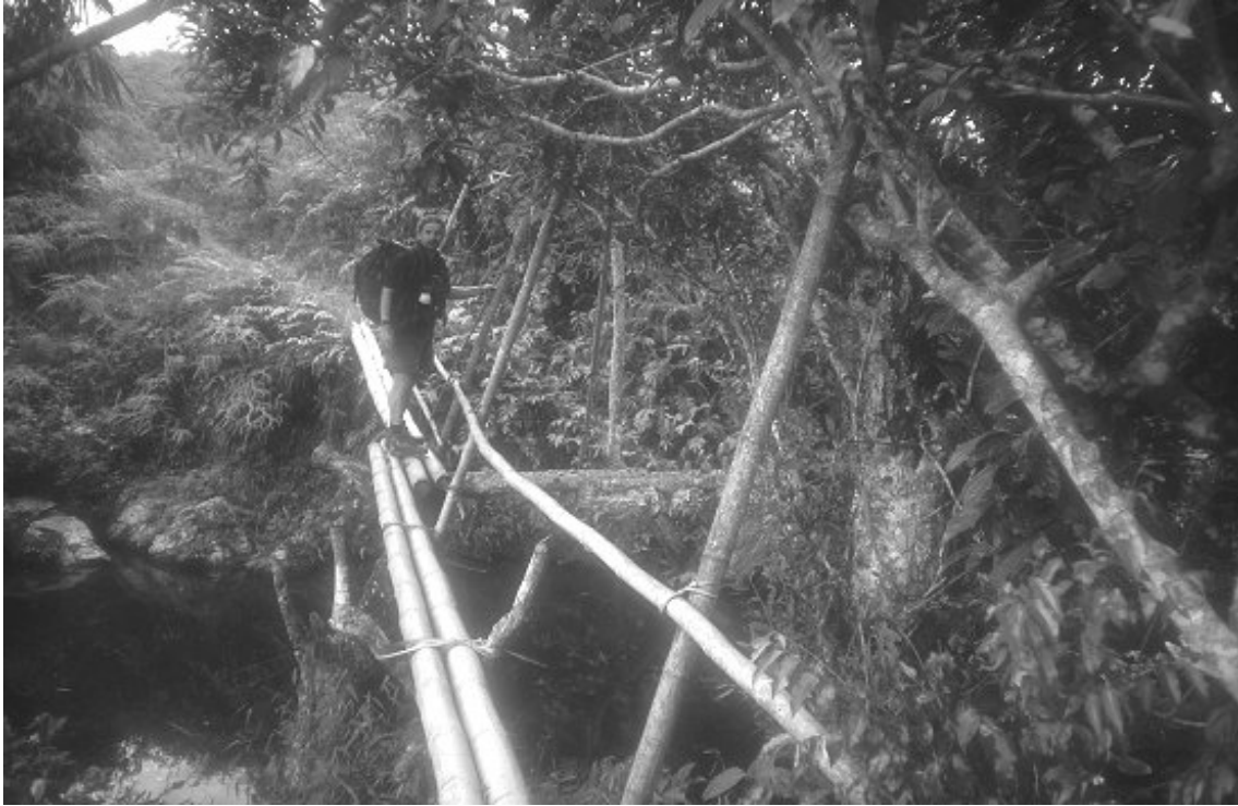
Figure 2.6. Crossing a bamboo bridge with handrails in Sabah. Photo: Bob Hartley©
