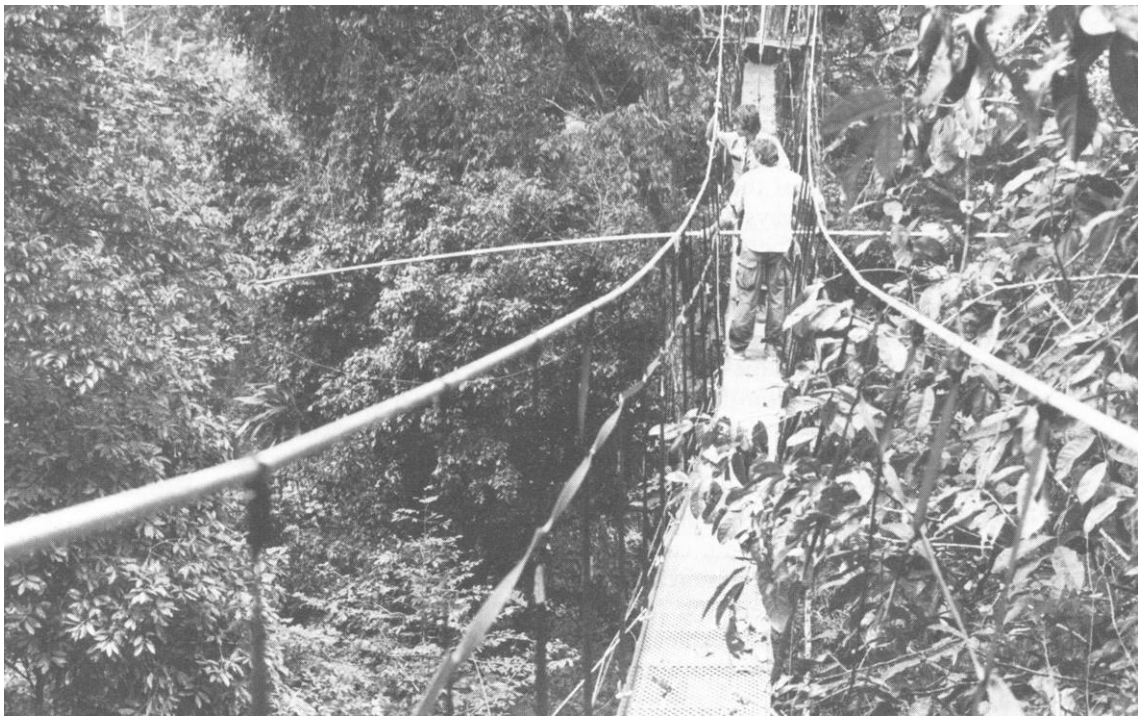
Figure 6.0 Telescopic clipper pole in use from Drake walkway, Panama. Rope main cables were later replaced with polyester tape. Photo: C. Sainsbury
